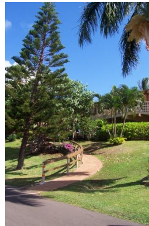
New Safety Railing between Units 136 & 137
